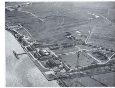
Southern sewage works
