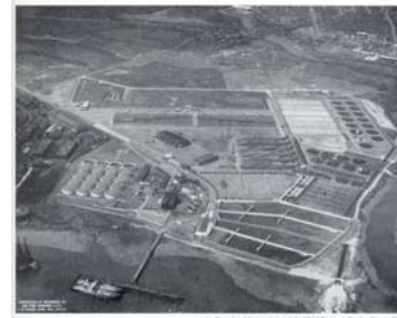
Northern sewage works
