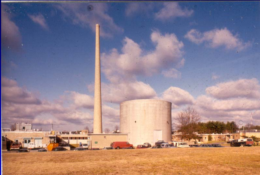
Brookhaven Medical Research Reactor
