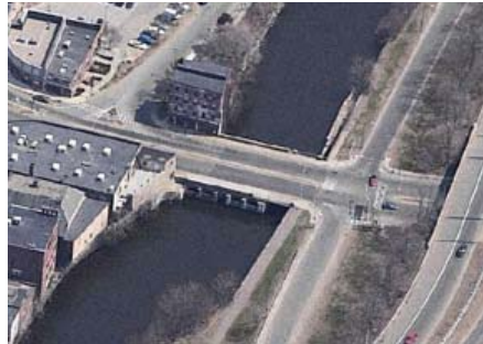
Aerial photo of the current configuration of Route 16 on and off ramps.
