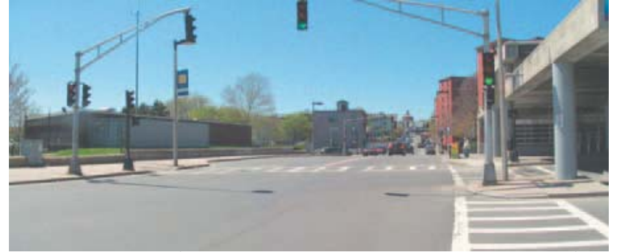
Figure 3: View of Existing Jackson Square
